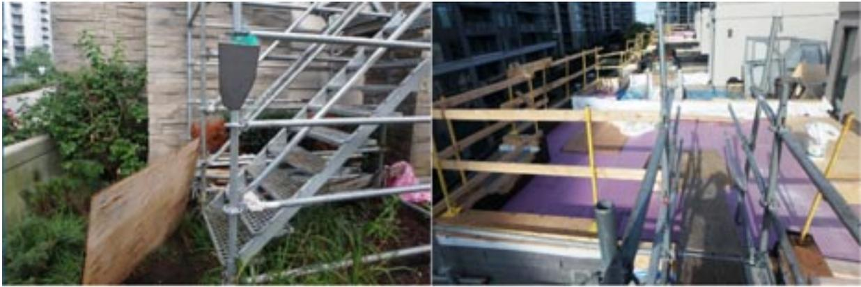
Figure 2 Scaffolding erected to enable the roof replacement project to proceed during the summer. Photo credit: RDH Building Science Inc.
